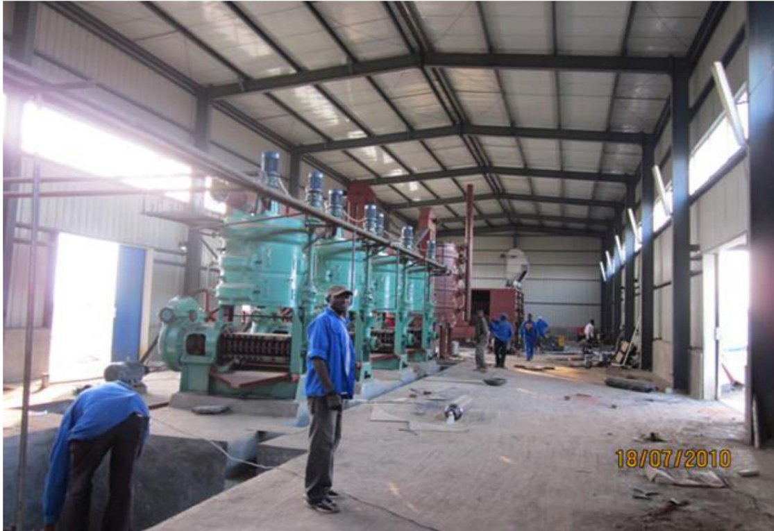
Oil Press Equipment being Installed in Sudan
